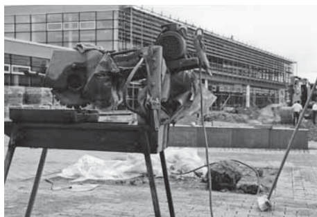
Baustelle Campus Rheinbach (1999).
